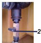
Fig. Pump system 1. Filter housing 2. Drain valve
